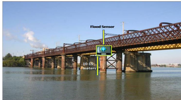
Figure 6 : Installed Flood Sensor
