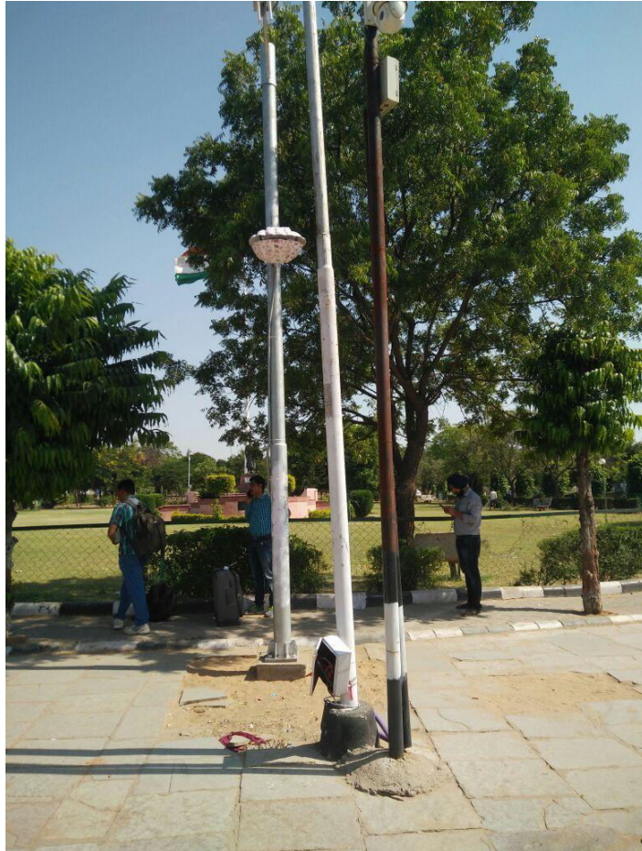
Figure 3 : Installed Environmental Sensor (Housing 1)
